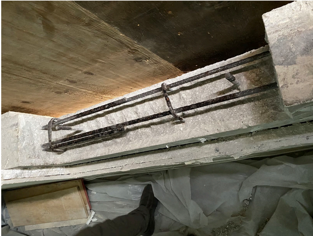
Picture 1: Unit 501 sill repair
