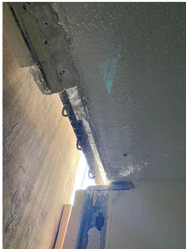
Picture 2: Unit 501 header repair
