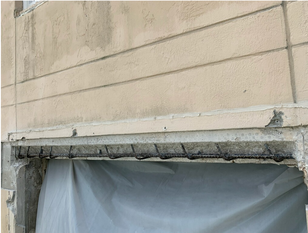
Picture 3: Unit 301 header repair
